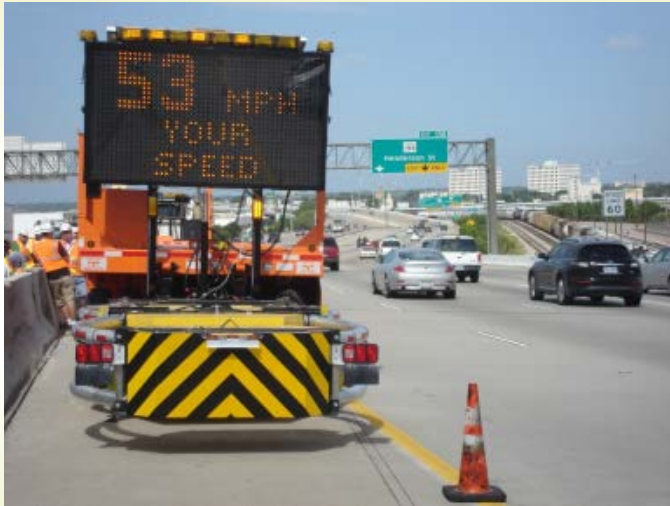
Signage w/ Radar
