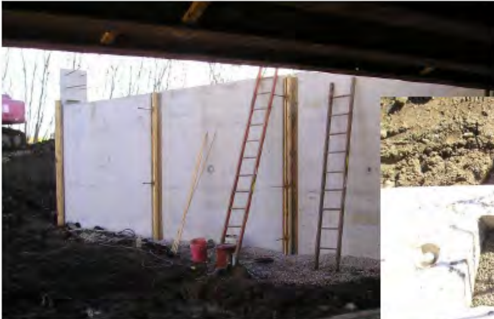
Form the vertical joint – shear key
