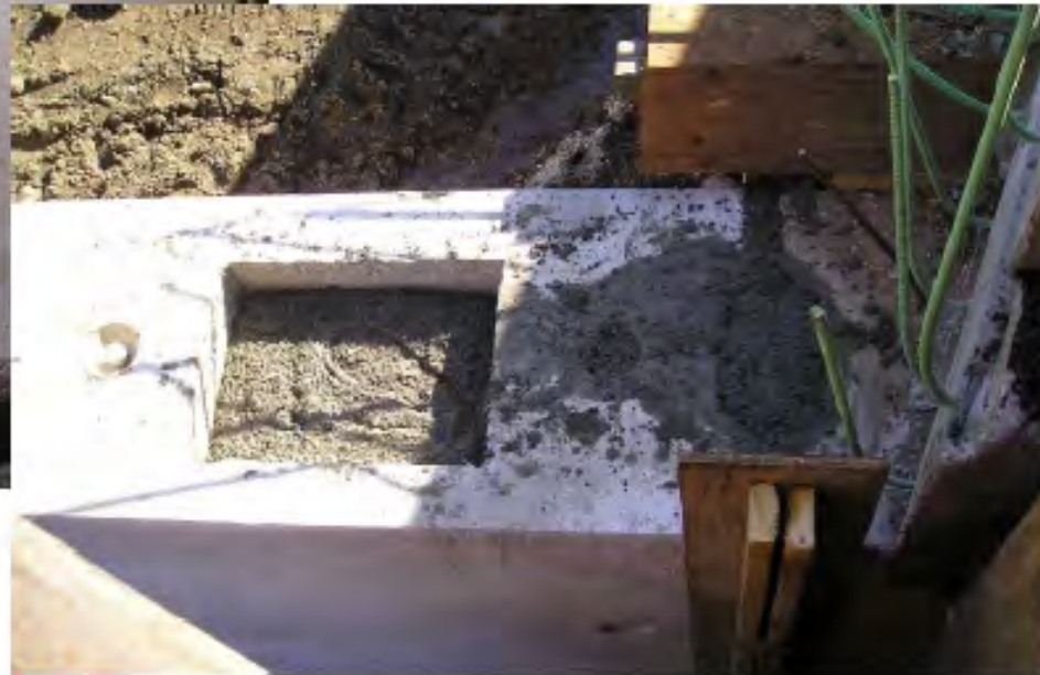
Grout the shear keys and pile block outs
