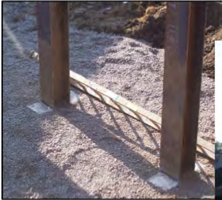
Drive the piles Weld the temporary supports
