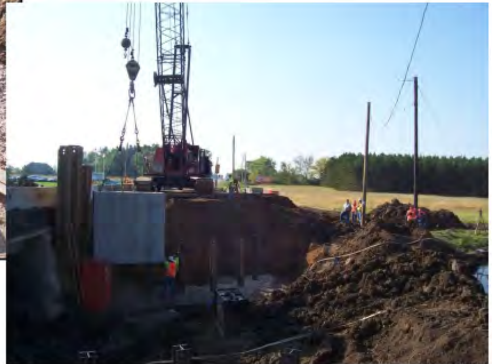
Erect the modules on Piles
