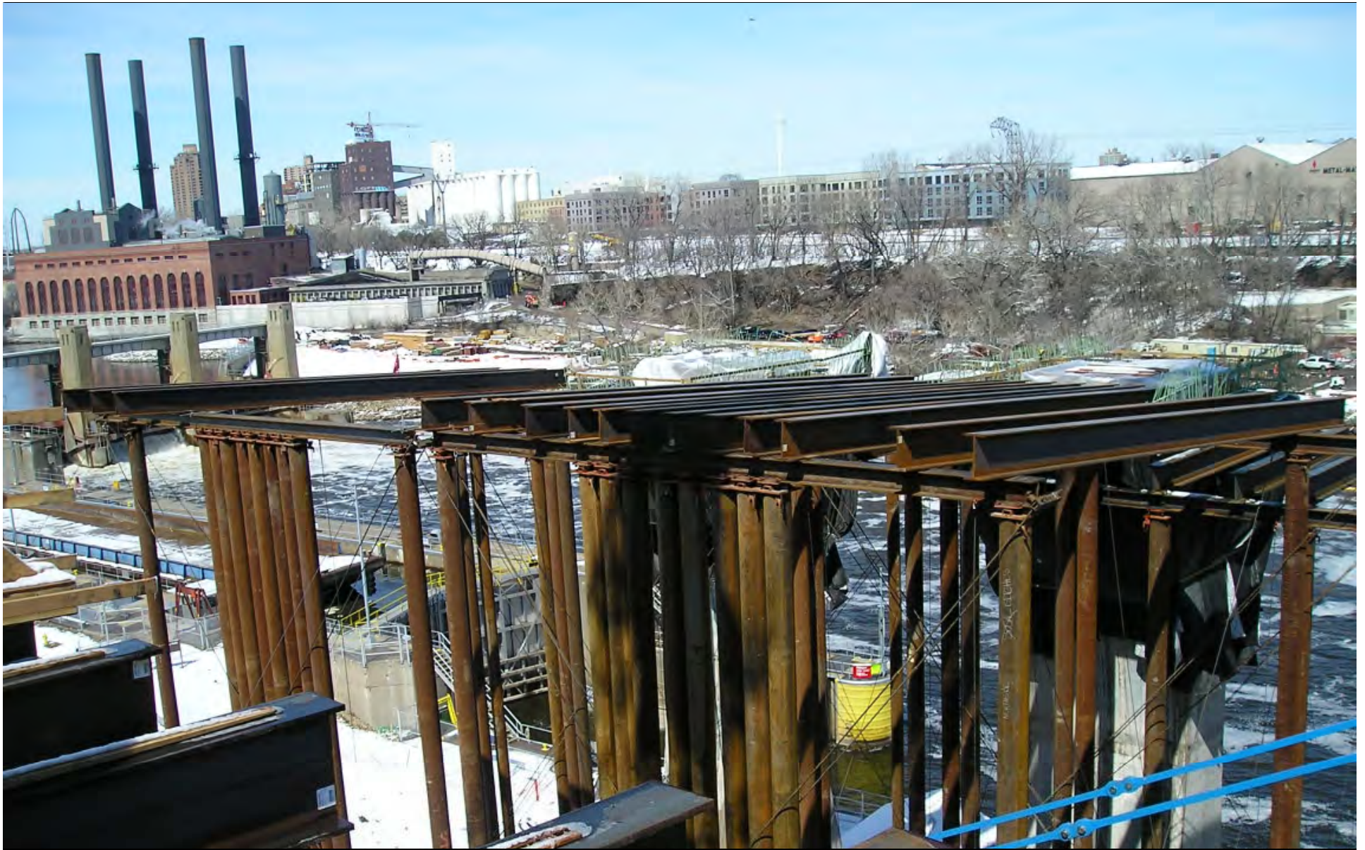
South side falsework
