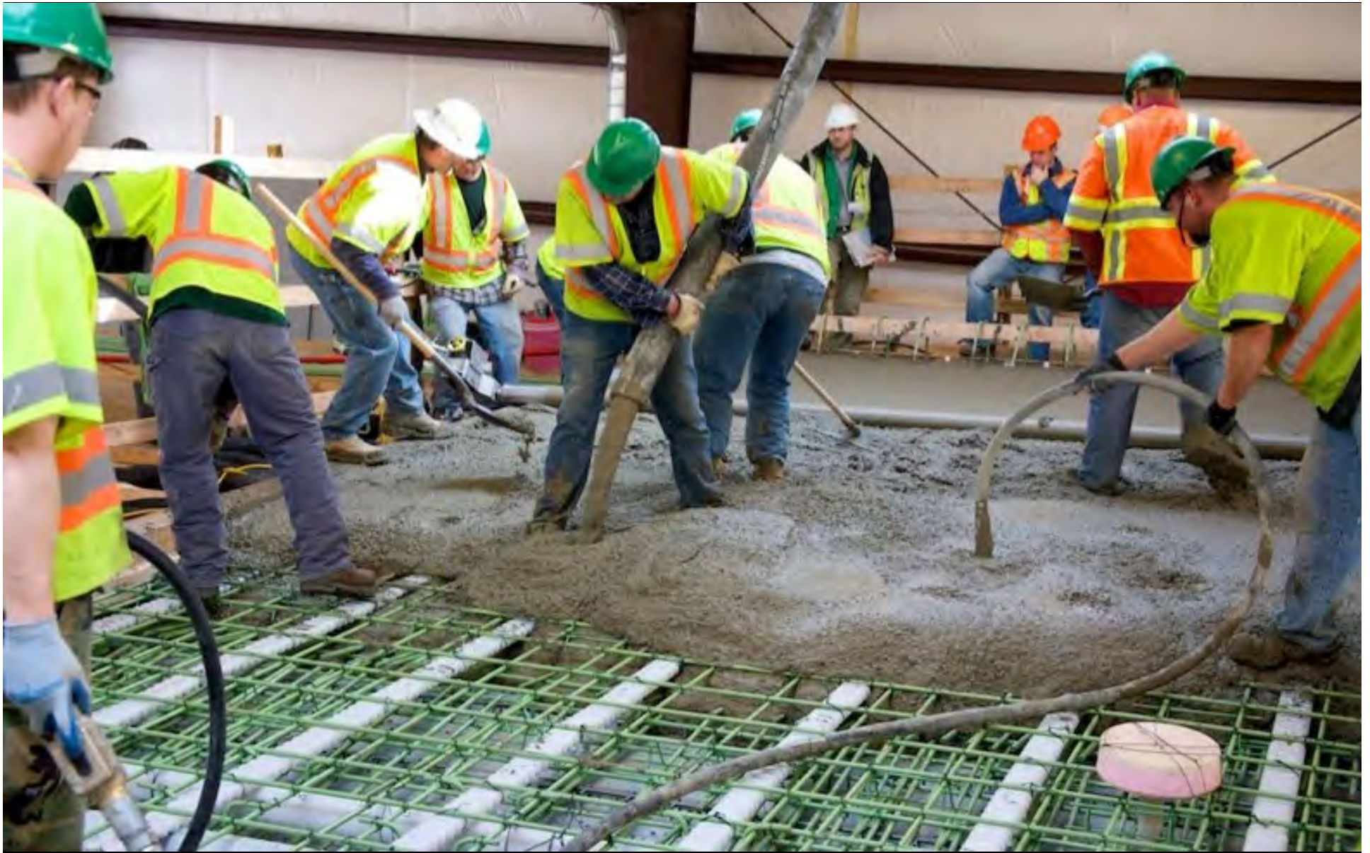
Pouring top slab, road bed, first segment, Feb. 19, 2008
